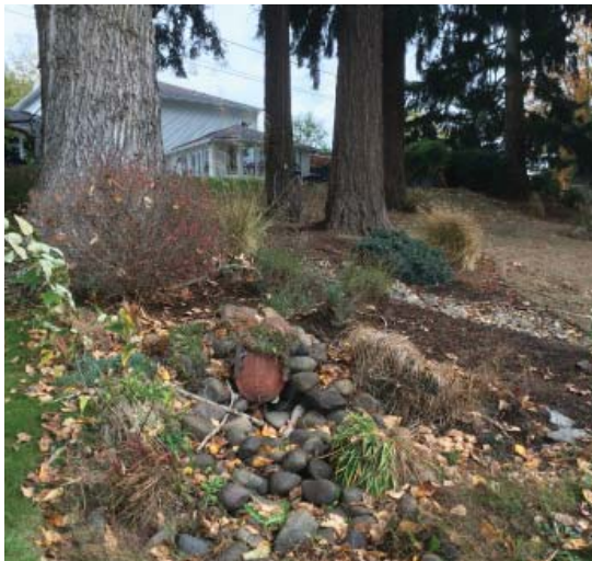
The existing outfall was directly under mature trees.
