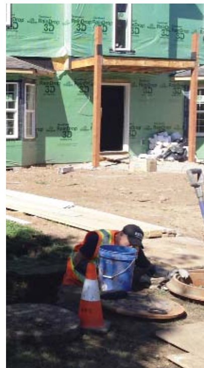
City crews first had to locate the manhole.
