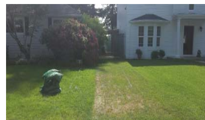
The home addition was completed before the storm drain could be relocated.
