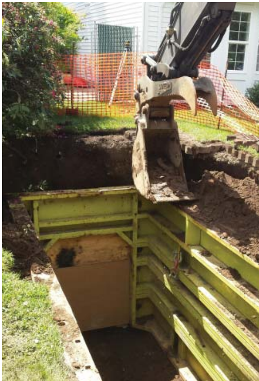
Shoring techniques were used to stabilize the excavated bore pit.
