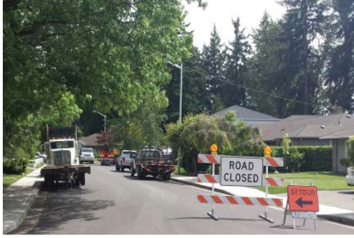
The road was closed to accommodate the construction equipment.
