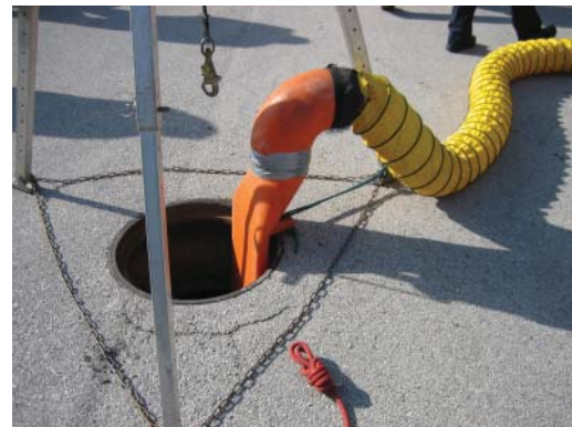
A Saddle Vent is a contoured durable plastic duct that allows workers to enter/exit a confined space without interrupting the ventilation.
